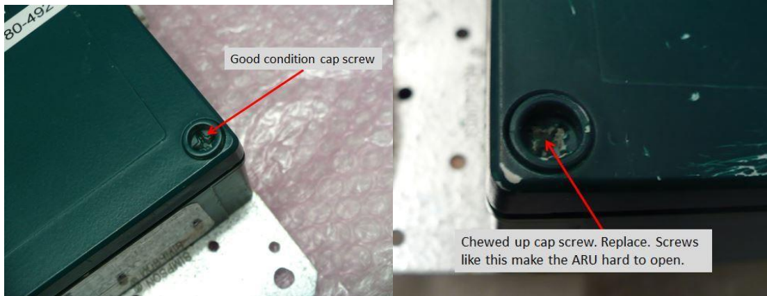
Figure 3: Examples of caps screws in good condition (left) and damaged condition (right).
